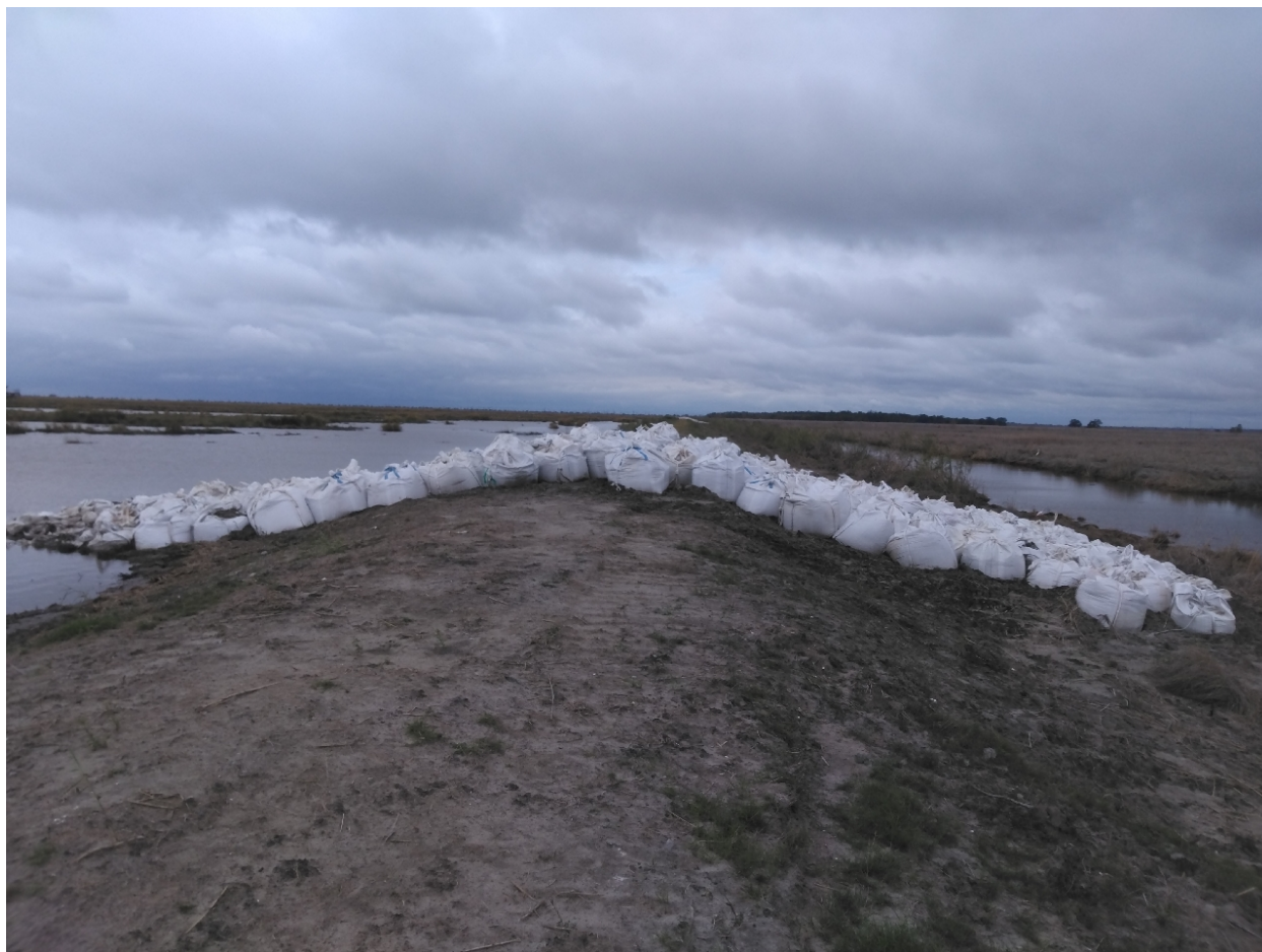
Figure 4. Overview of Levee cut #7b taken along the levee (view north; 22 Nov 2021). Excavator track marks were generally restricted to the levee footprint.
